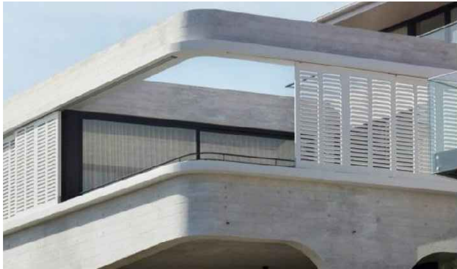
timber shutters(white painted)
