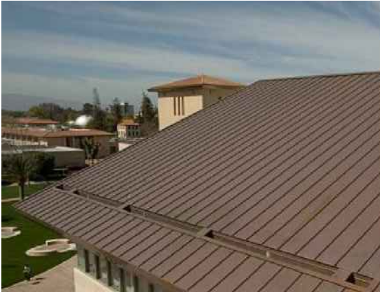
metal roof sheeting (copper)
